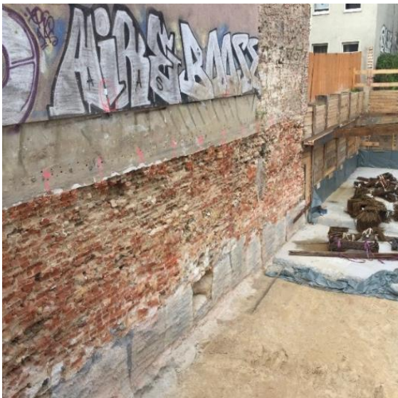
Figure 2 Underpinning existing foundation
