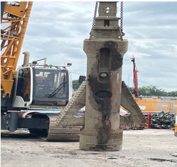
Figure 1. Pile base cutter in operation
