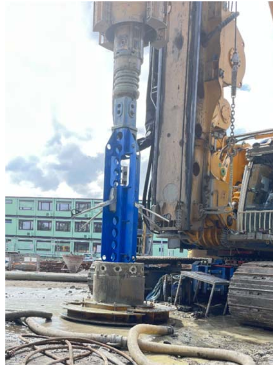
Figure 8: Kelly mounted pile inspector
