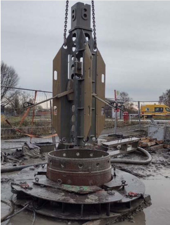
Figure 9: Service crane mounted pile inspector
