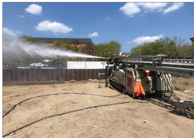
Fig.3: High power beam released from a jet grouting rig
