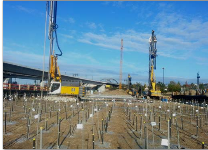
Fig.2: View over the injection tubes
