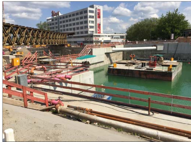
Fig.4: Working ponton for divers
