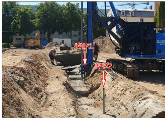
Fig.12: Test set- up while measuring the diameter of the cured column
