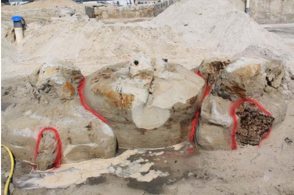
Figure 10: excavated test columns
