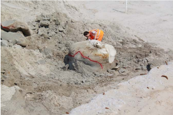
Figure 11: excavated primary column
